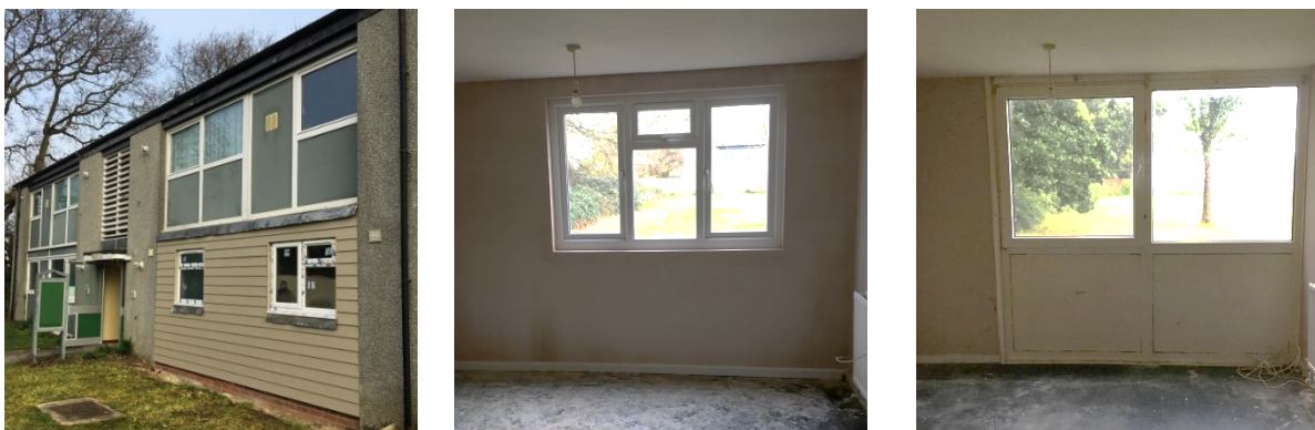
Left to right: Pilot project – PVC-u panel prior to works, wall and window following works, frontage following works (bottom)
